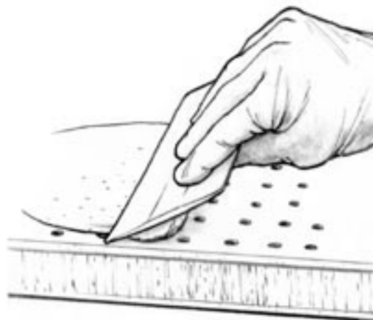
Figure 5-4 Fill any remaining voids and fair the surface with an epoxy/407 mix.
