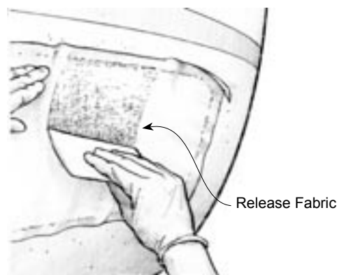
Figure 4-6 Squeegee over the release fabric with firm pressure to remove excess epoxy and smooth the patch.
